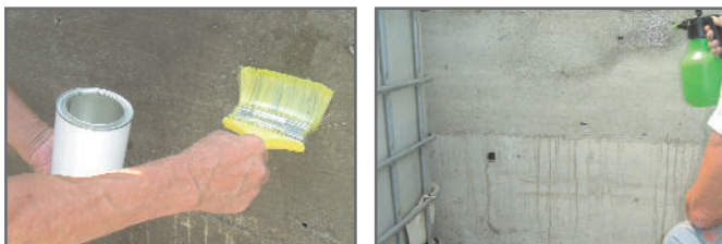
The highly absorbent substrates must be primed or very porous with connecting bridge AT RESINOV or AT EPO REX.
