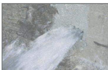
1. Clean around the leak to allow the product to anchor on firm surface.
