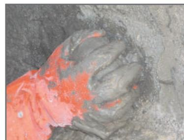
3. Seal the leak, keeping the pressure until the product takes effect and repeat if necessary.
